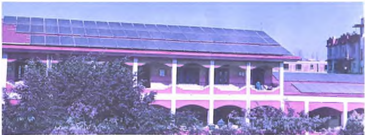
Fig. 7: Roof top on grid solar panel, K.C. Das Commerce College
